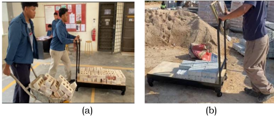
Figure 9:(a) Workability test in brickwork workshop, (b) Workability test at construction site
