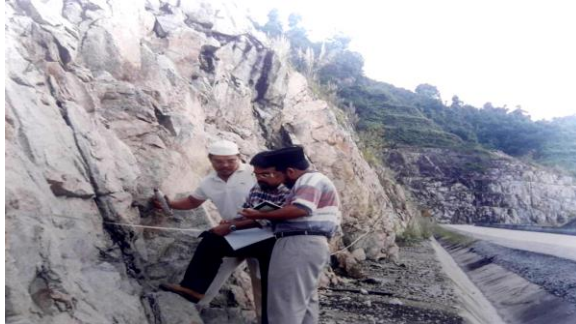
Picture 3: Measurement of fracture distance. Measuring tape is used to determine the distance between fracture section
