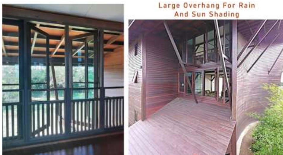
Figure 10: Large overhang of Anjung Kelana
